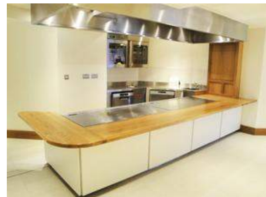
In-built serving counter
